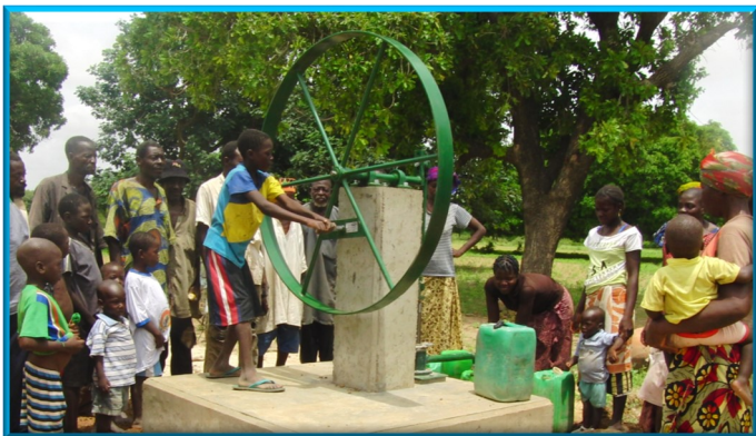
2019: 38 water pumps and 38 wells, new or fixed.
